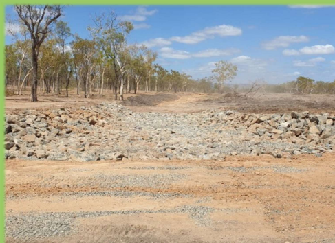
Active head of gully (gully is approximately 3km in length and up to 2m in depth) and completed rock chute on the gully head November 2020
